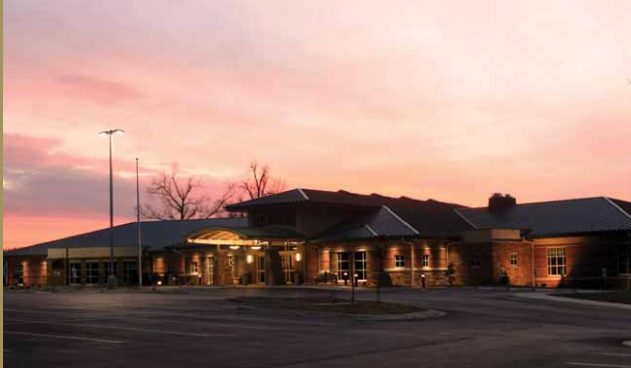
The new, Donald W. Reynolds Library at sunset.
